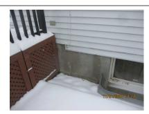
**LOCATION:** Throughout **SYSTEM:** Exterior **CONDITION:** Grading near foundation has settled
