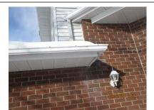
**LOCATION:** Various Locations **SYSTEM:** Roof **CONDITION:** Downspout discharges onto lower roof surface
