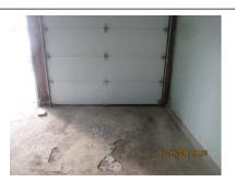
**LOCATION:** Garage **SYSTEM:** Exterior **CONDITION:** Garage concrete floor is damaged.
