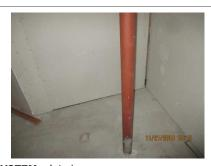
**LOCATION:** Basement on edge of floor **SYSTEM:** Interior **CONDITION:** Evidence of prior leak in exterior wall; suspected
