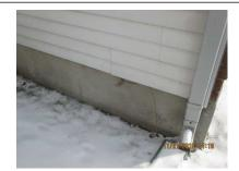
**LOCATION:** Various Locations **SYSTEM:** Roof **CONDITION:** Downspout discharges too close to house
